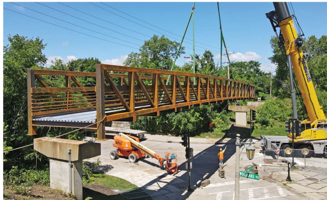
Woodland Pedestrian Bridge
